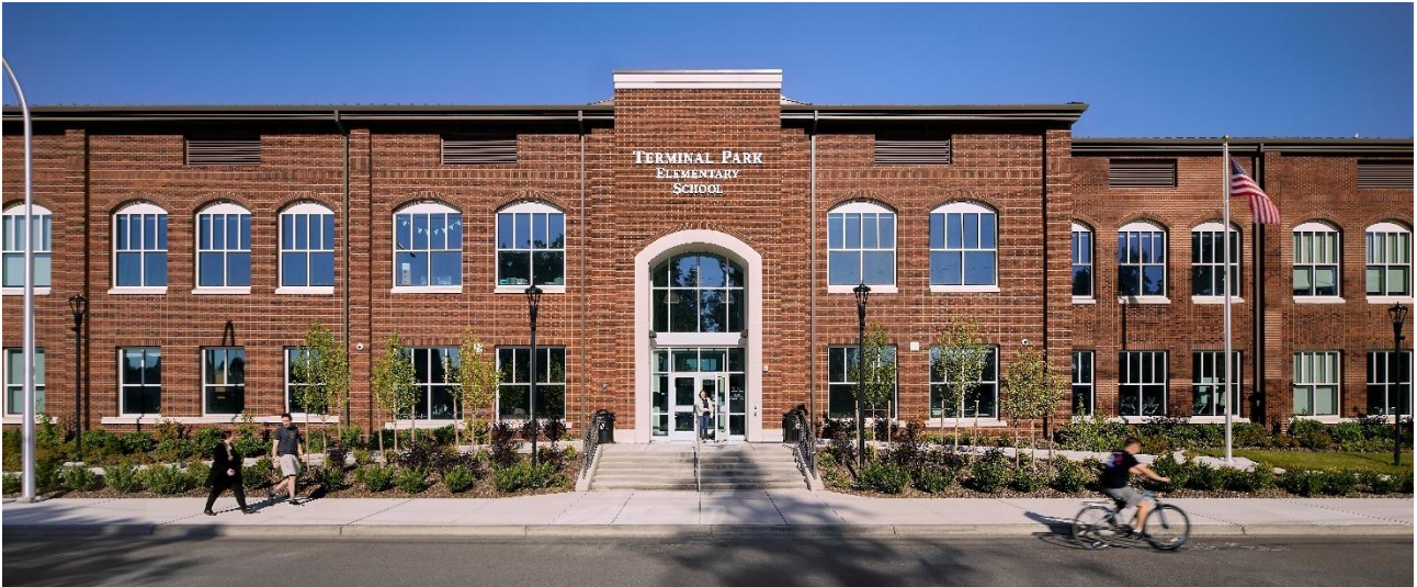
Terminal Park Elementary School – 2023
